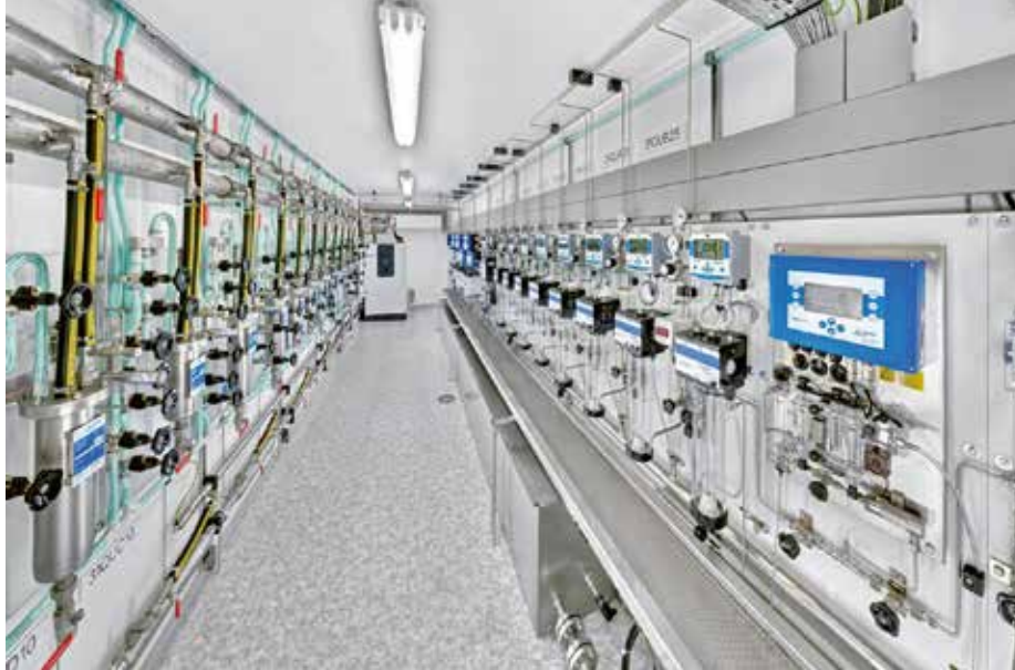
SWAS container with separated conditioning analysing part
