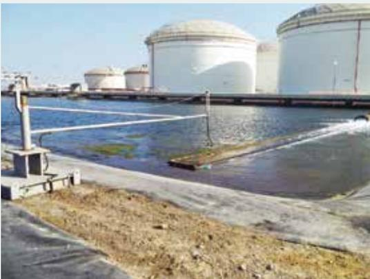
Fuel fired power generation plants have several Leakwise ID-223 Oil Sheen Detectors installed in oil and storm water collecting sumps, and separators/interceptors located in containment area near tanks. These sumps need to be monitored for safety and environmental purposes. Leakwise sensors can also
