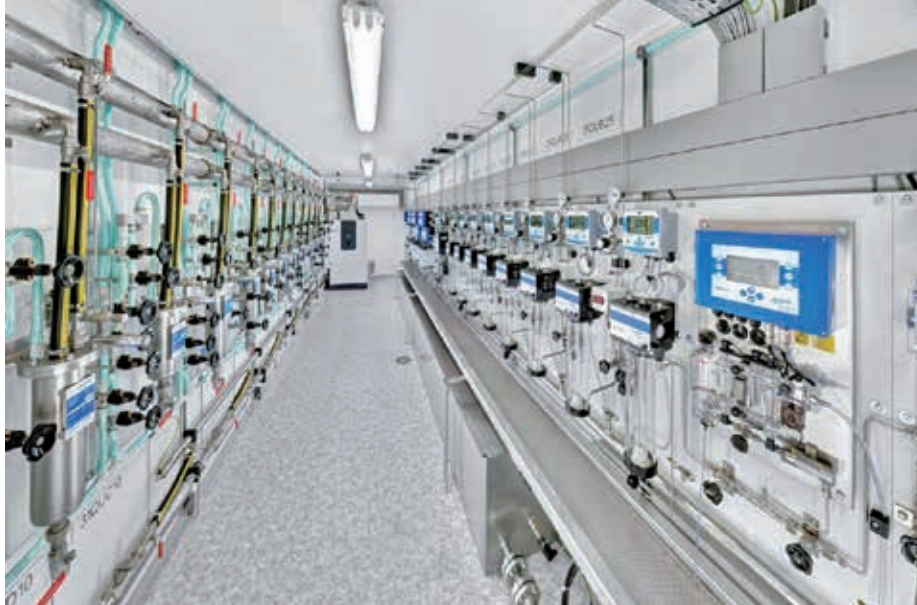
SWAS container with separated conditioning analysing part
