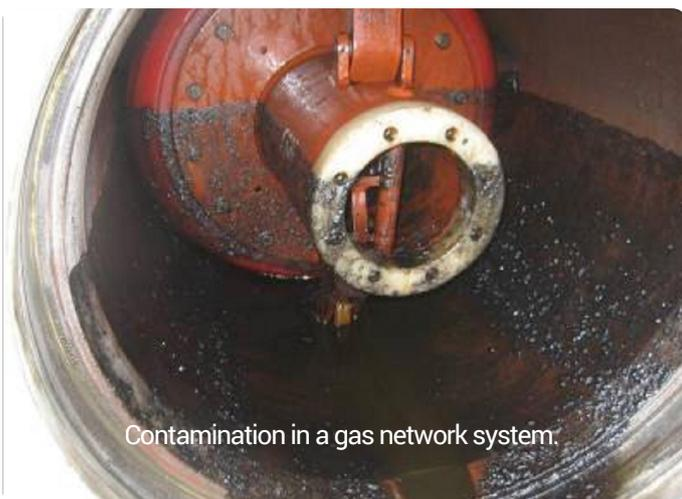
Contamination in a gas network system.
